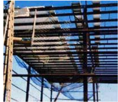
A safety net is being used under the roof of this building as an acceptable fall protection system.
