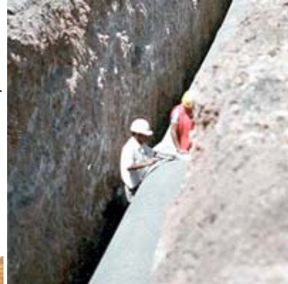
These workers are not protected from a cave-in, nor do they have any apparent safe access or egress from the trench.
